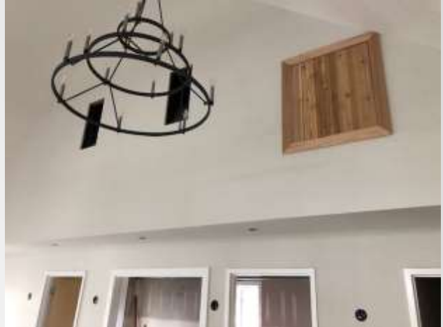
Hatch door to match the beams in the upper storage area
